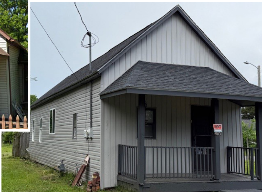
503 Walter Jetton after participating in the Home Repair Micro Grant
